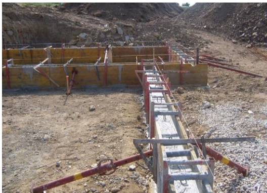
beton in bekisting
