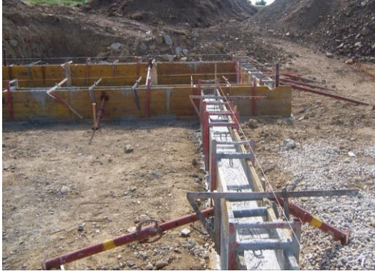
beton in bekisting
